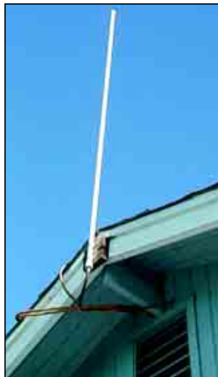
Figure 5—The completed antenna mounted to the roof.
